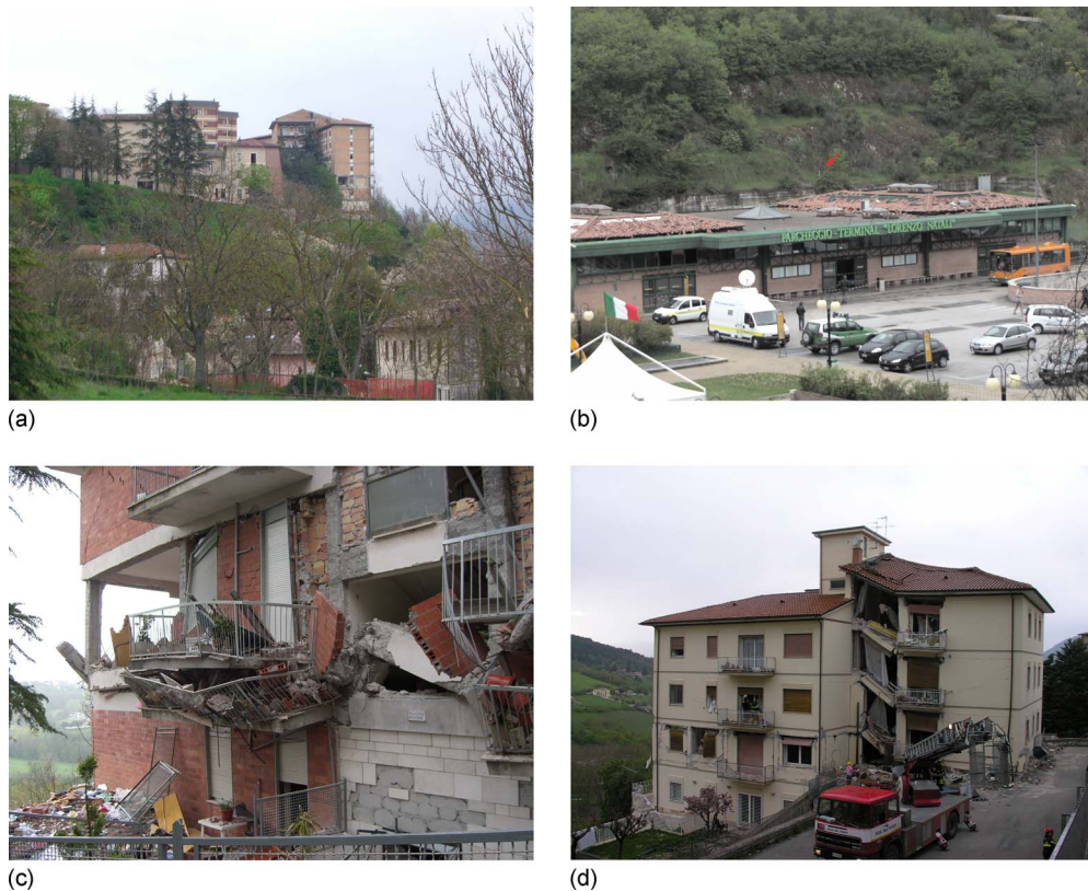
Figure 9. Cases where topographical effects may have played a role influencing the shaking imposed on these buildings. (a) A building with damages to the infill walls. (b) The bus depot behind which there is a retaining wall above which station AQK is housed. Arrow shows GPS antenna of the station. (c) Via Gualtieri d'Ocra, L'Aquila: mid-story pancake collapse, (d) another partial collapse of a building founded on a slope.
