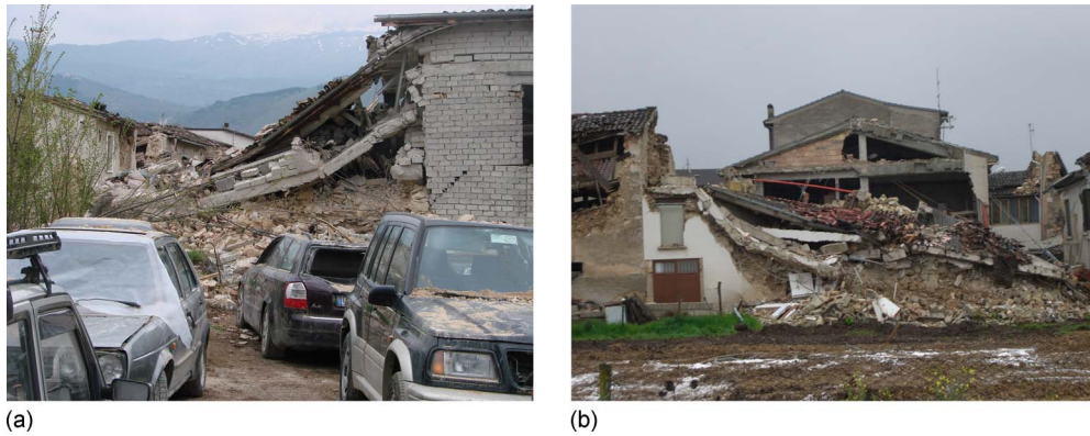
Figure 7. A majority of buildings in Onna (MCS 9.5 according to Galli and Camassi 2009 ). Mostly older, poor, nonductile masonry and un-engineered suffered heavy damage or collapsed.
